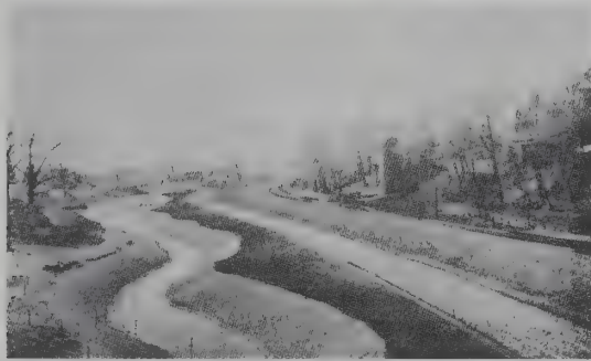
The Riverway, Boston, ca 1892, showing graded embankments ready for planting. To the right, a mound separates the park from a recently installed trolley line. (Below) Approximately thirty years after construction, having achieved a wholly "natural" appearance, the adjacent trolley line now hidden behind mound and plants. Project was primarily for flood control.
